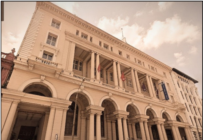
Image courtesy of Google Street View.
