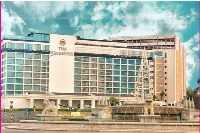
Image courtesy of The Kingsbury Hotel.
